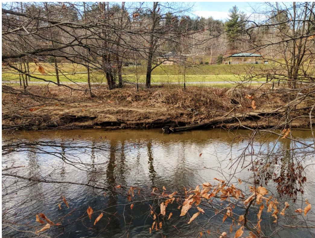
< River left erosion near Brookshire Park loop
