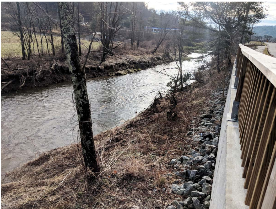
Active erosion along Town owned River right streambank
