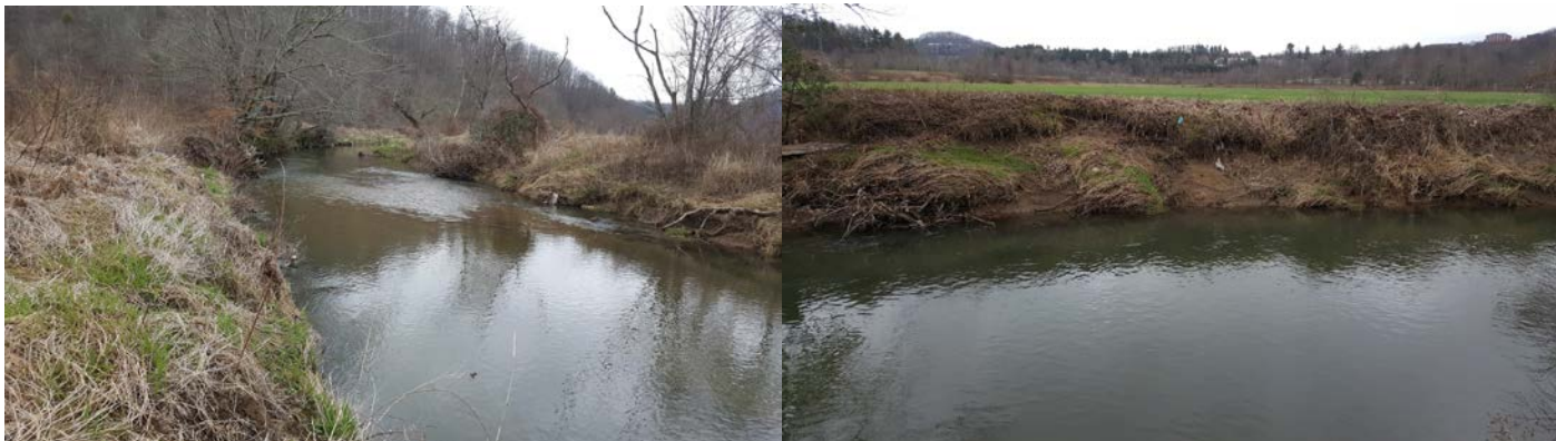
(Left) Before construction, the river had no access to the existing floodplain. (Right) Before sloping, the banks were actively eroding and lacked any woody vegetation.
