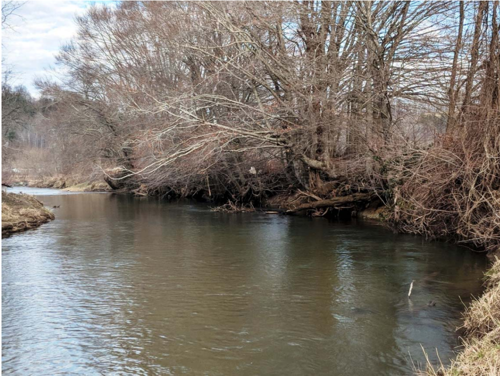
< Eroding river left stream bank along Watauga County property. Leaning trees.
