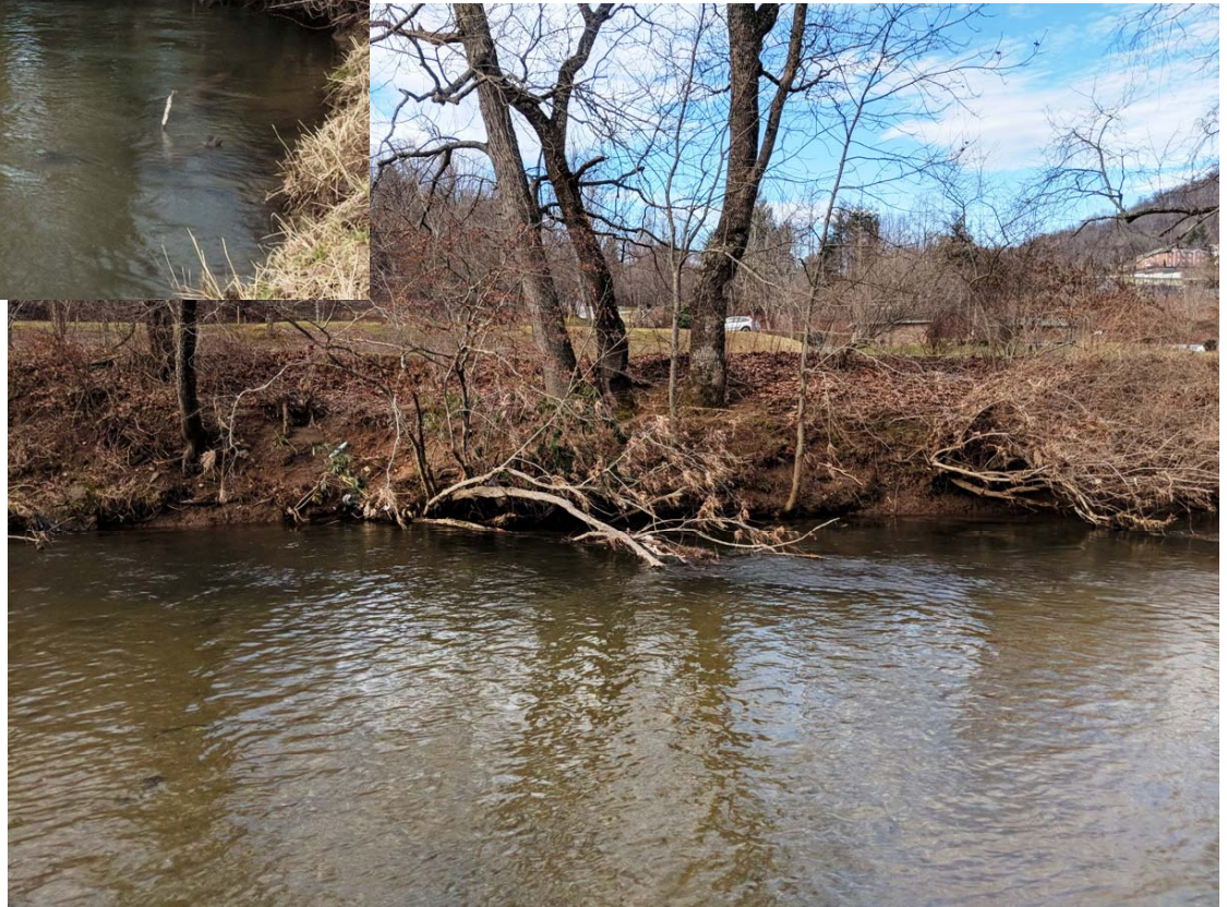
Eroding river left streambank Near asphalt trail >
