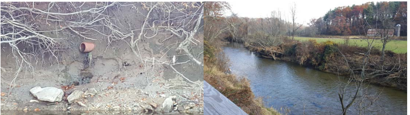
(Left) A terracotta drainage pipe from historic agricultural landuse sticks out of the river bank from erosion. (Right) Vertical streambanks with little to no vegetated buffer.
